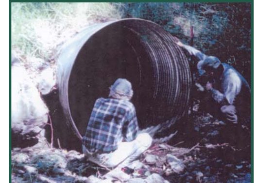
Figure 2: Assessing the condition of a culvert in Lobster Creek in 1998
