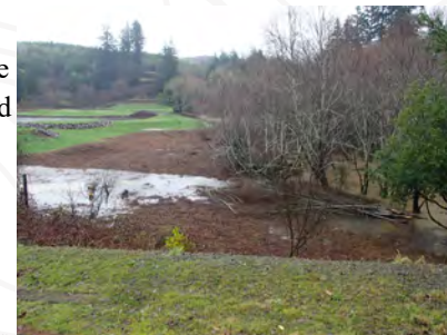
Pulling this orphaned road crossing on Jack Creek will restore access to a 2-acre wetland.
